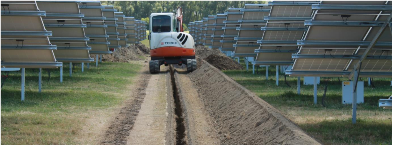
Plate 15.18: Cabling Channels during Cable Installation
